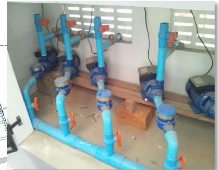
Water meter installation
