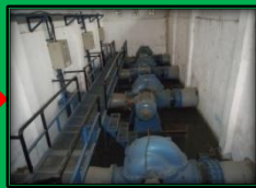
Low lift pumps
