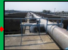
Rapid sand filter
