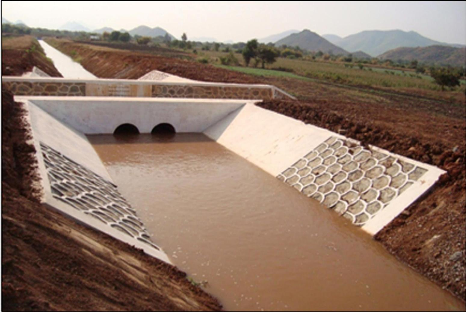
Drainage Crossing at Weir Right Main Canal, RD-13+400'
