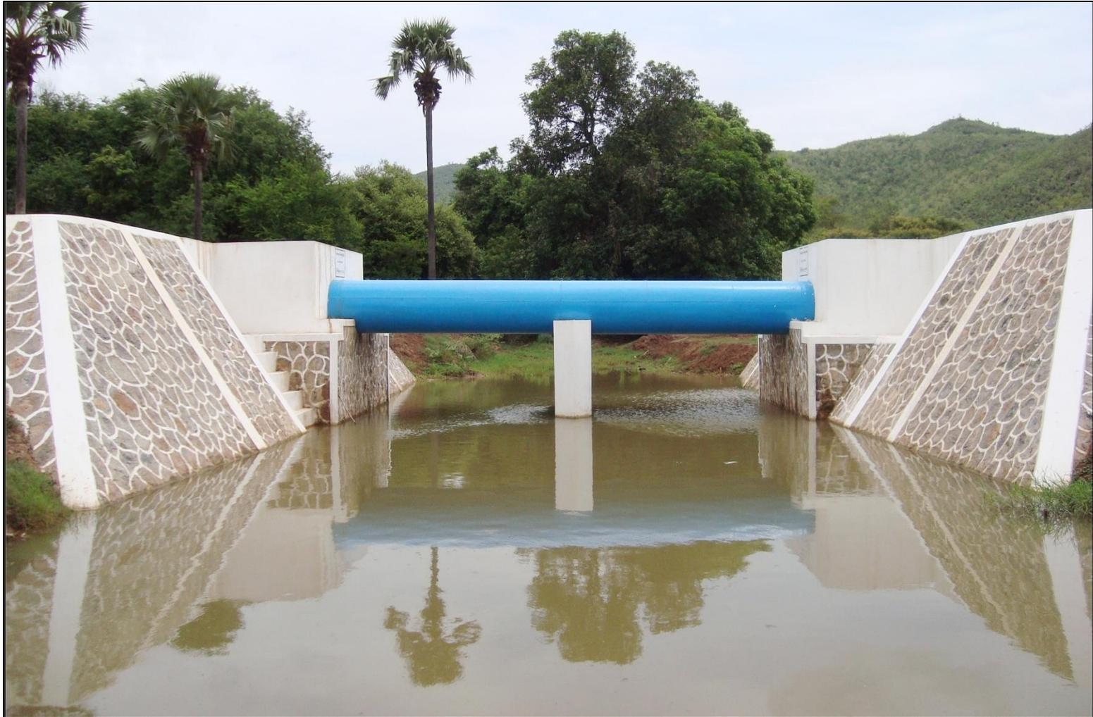
Drainage Crossing at Weir Left Main Canal, R.D-94+50'
