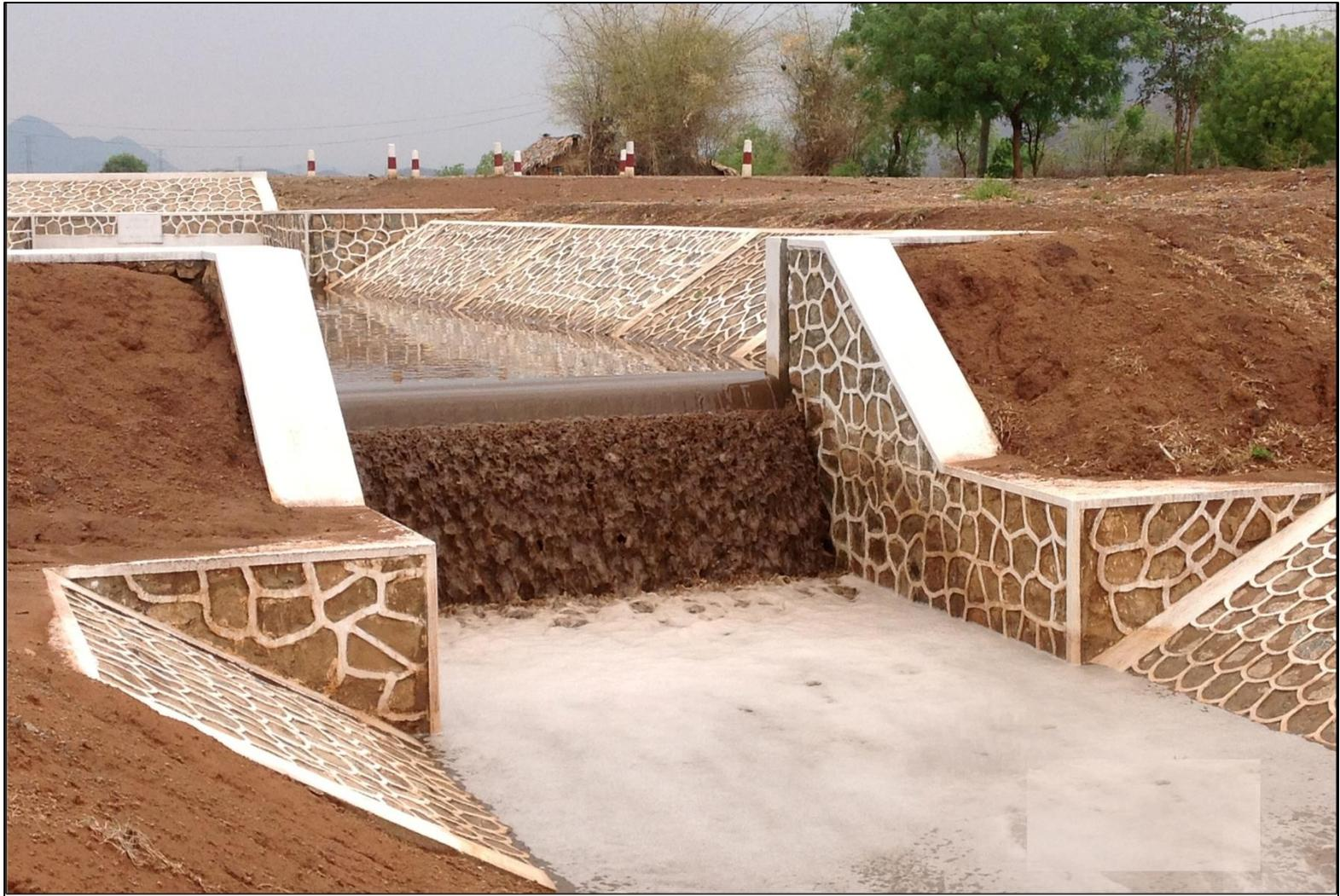
Drop Structure at Weir Left Main Canal, R.D 55+00'
